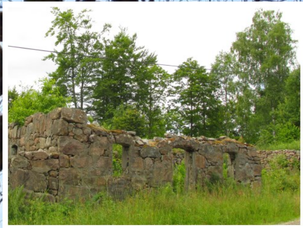
Gårdsruin, Jonsnahult / Farm Building Ruin, Jonsnahult
